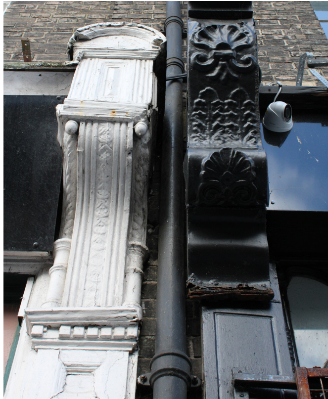
Fig. 048 Victorian console brackets.
