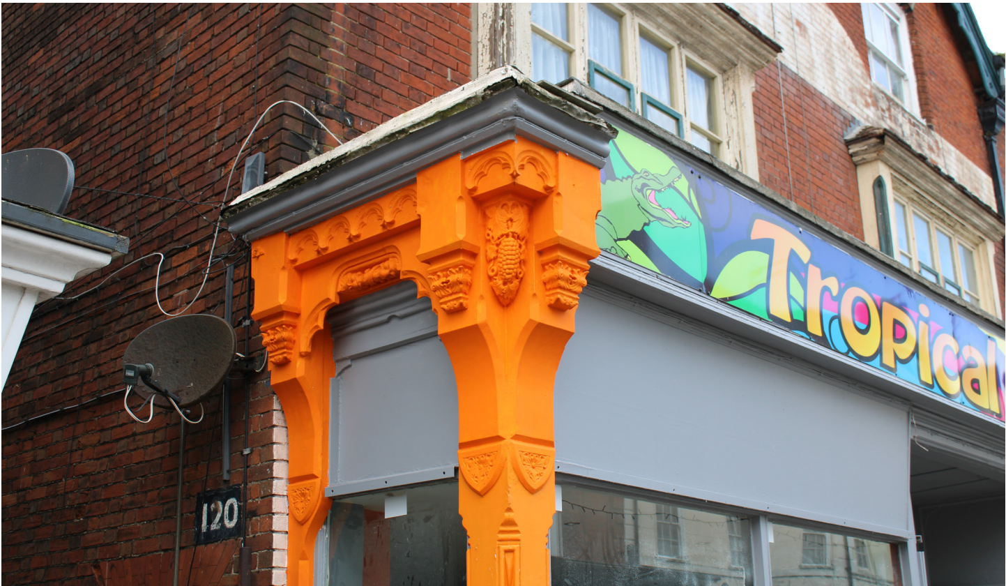
Fig. 012 Late Victorian console brackets, part of an unsympathetically treated historic shopfront on King Street, Great Yarmouth.
