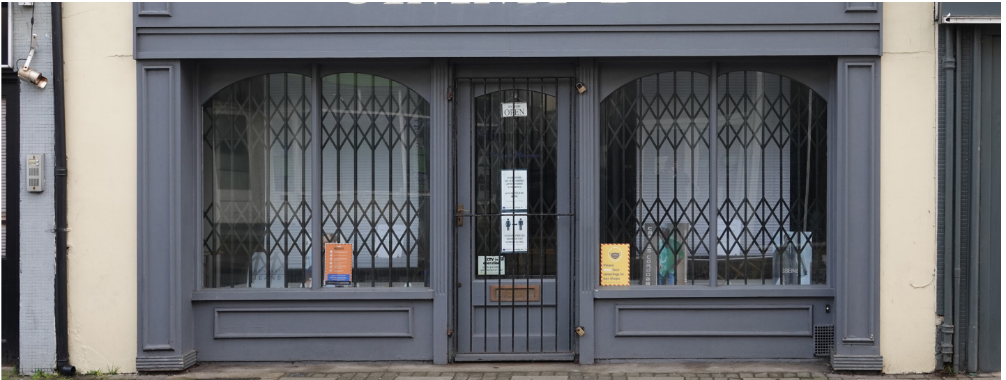
Fig. 054 Internal open lattice grilles.
