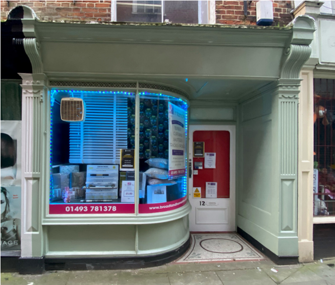
Fig. 032 Timber panelled stallriser.
