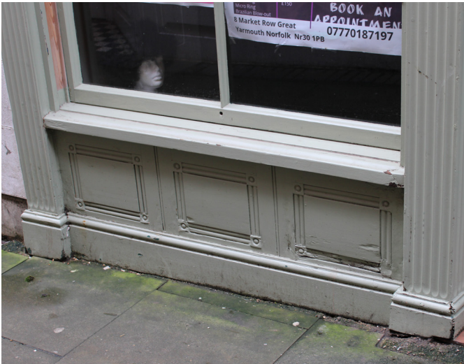
Fig. 033 Timber panelled stallriser.
