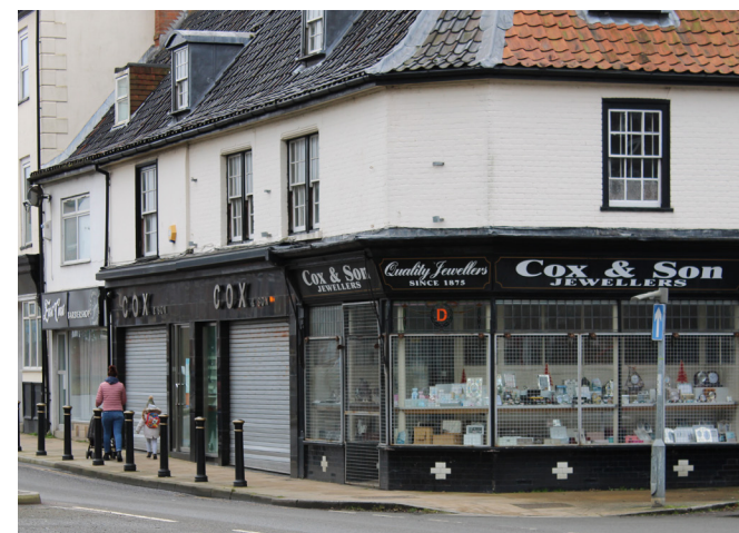
Fig. 045 Fascia angled towards the street - a traditional approach.
