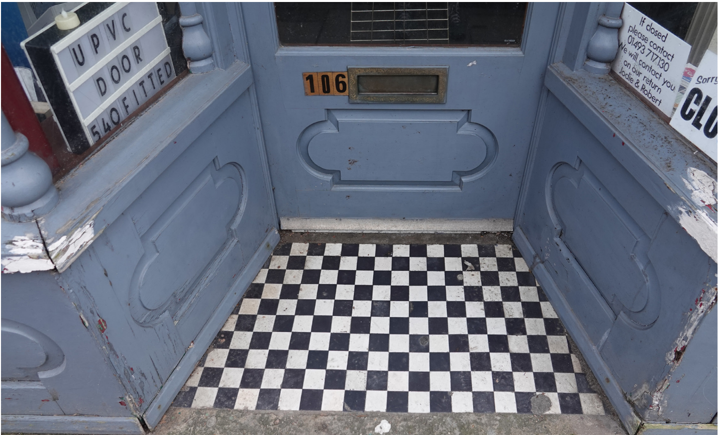
Fig. 038 Entrance lobby tiled in chequerboard pattern.
