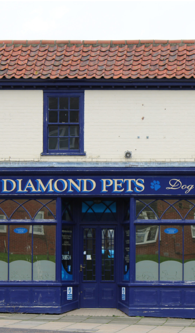
Fig. 041 Shopfront entrance - recessed doors with fanlight in line with the transom lights.
