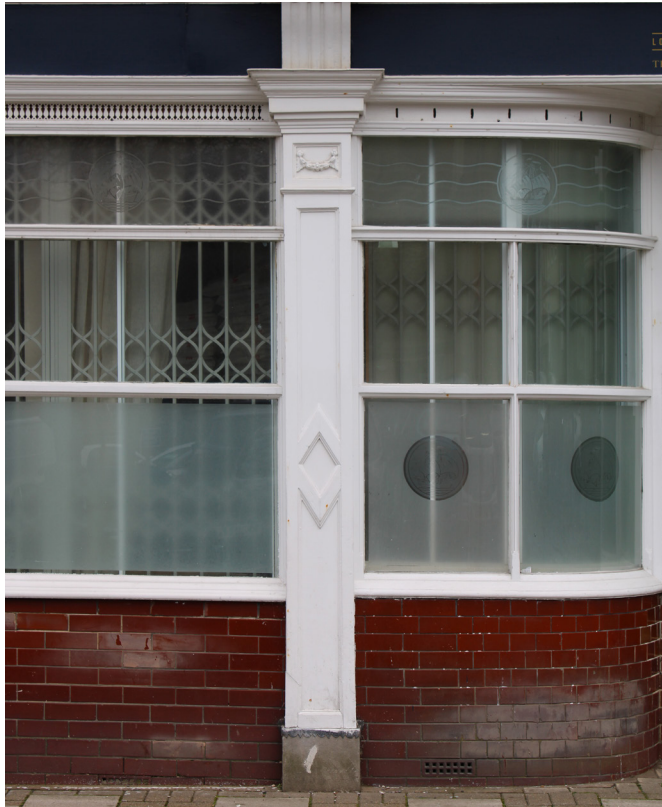
Fig. 047 Edwardian pilaster.
