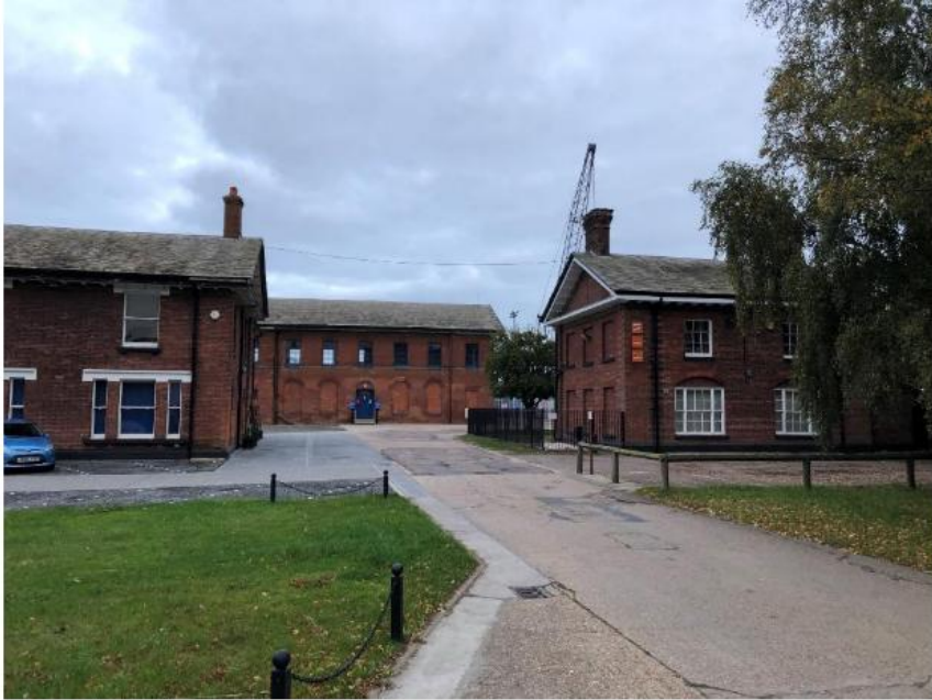
Figure 3 - 244 and 244b Southtown Road
