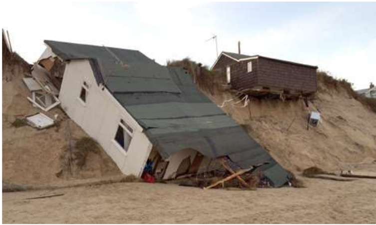
Figure 9 More recent erosion (2013) has caused further loss of properties. Near-vertical dune faces have formed during the storm events, undermining the chalets.
