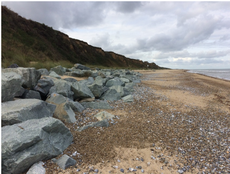
Figure 1 California rock berm
