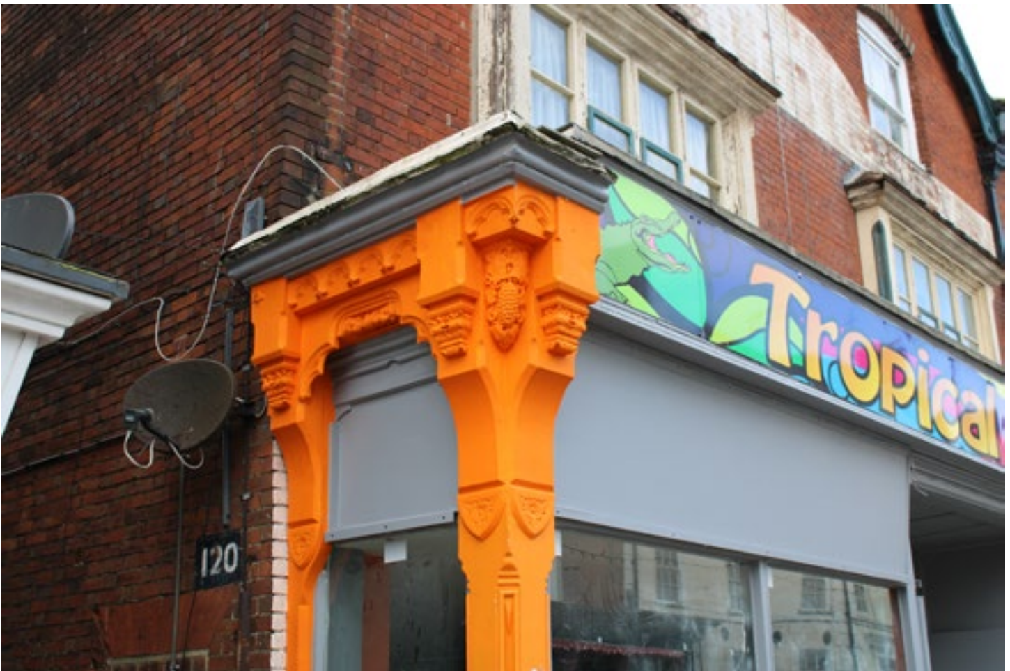
Fig. 014 Late Victorian console brackets on King Street, Great Yarmouth
