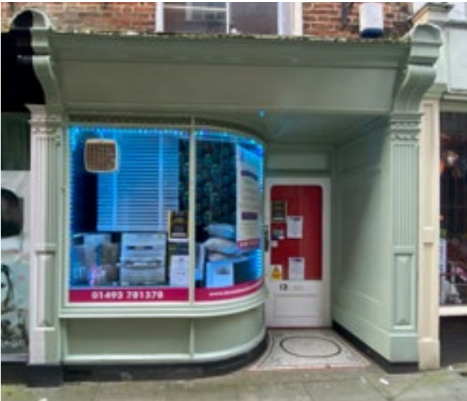
Fig. 026 Timber panelled stallriser
