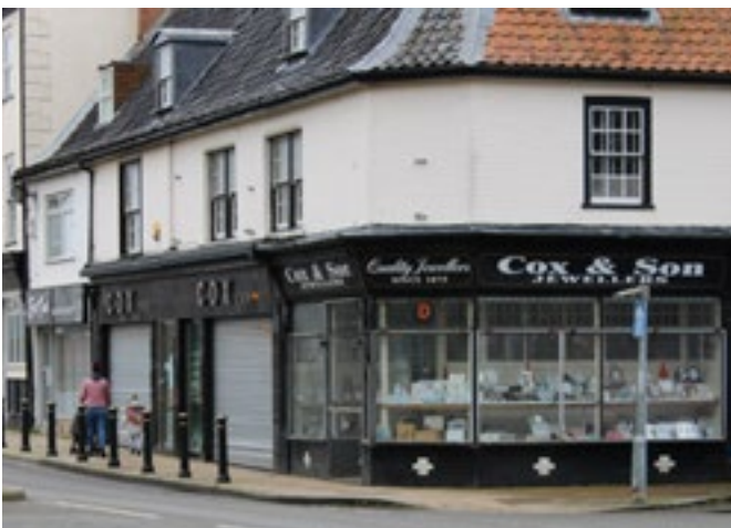
Fig. 039 Fascia angled towards the street - a traditional approach.
