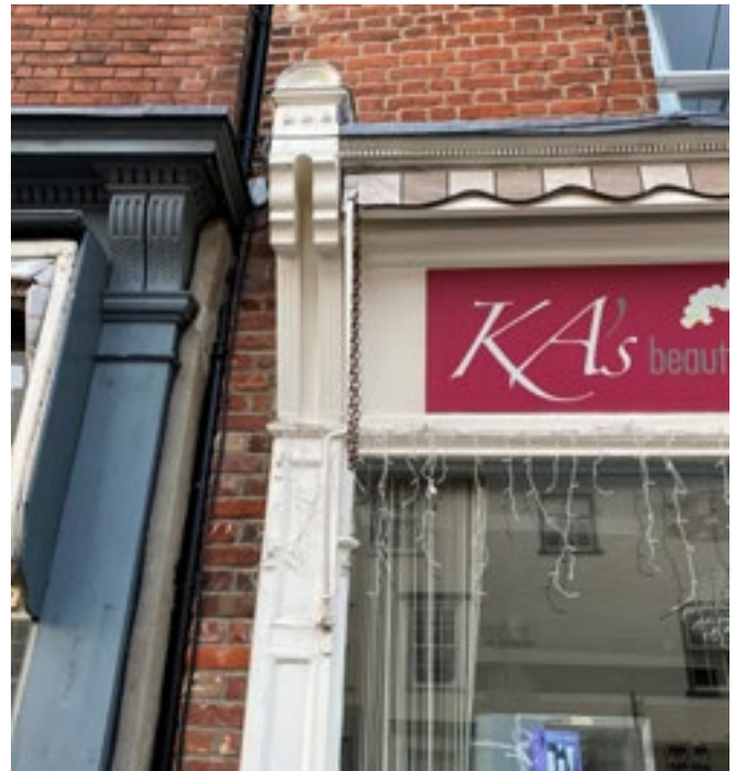
Fig. 049 Integrated blind box with a sprung roller housing a retractable canvas awning. Metal arms allow the blind to extend out and storm chains prevent movement.
