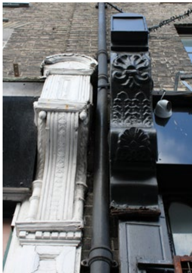
Fig. 042 Victorian console brackets
