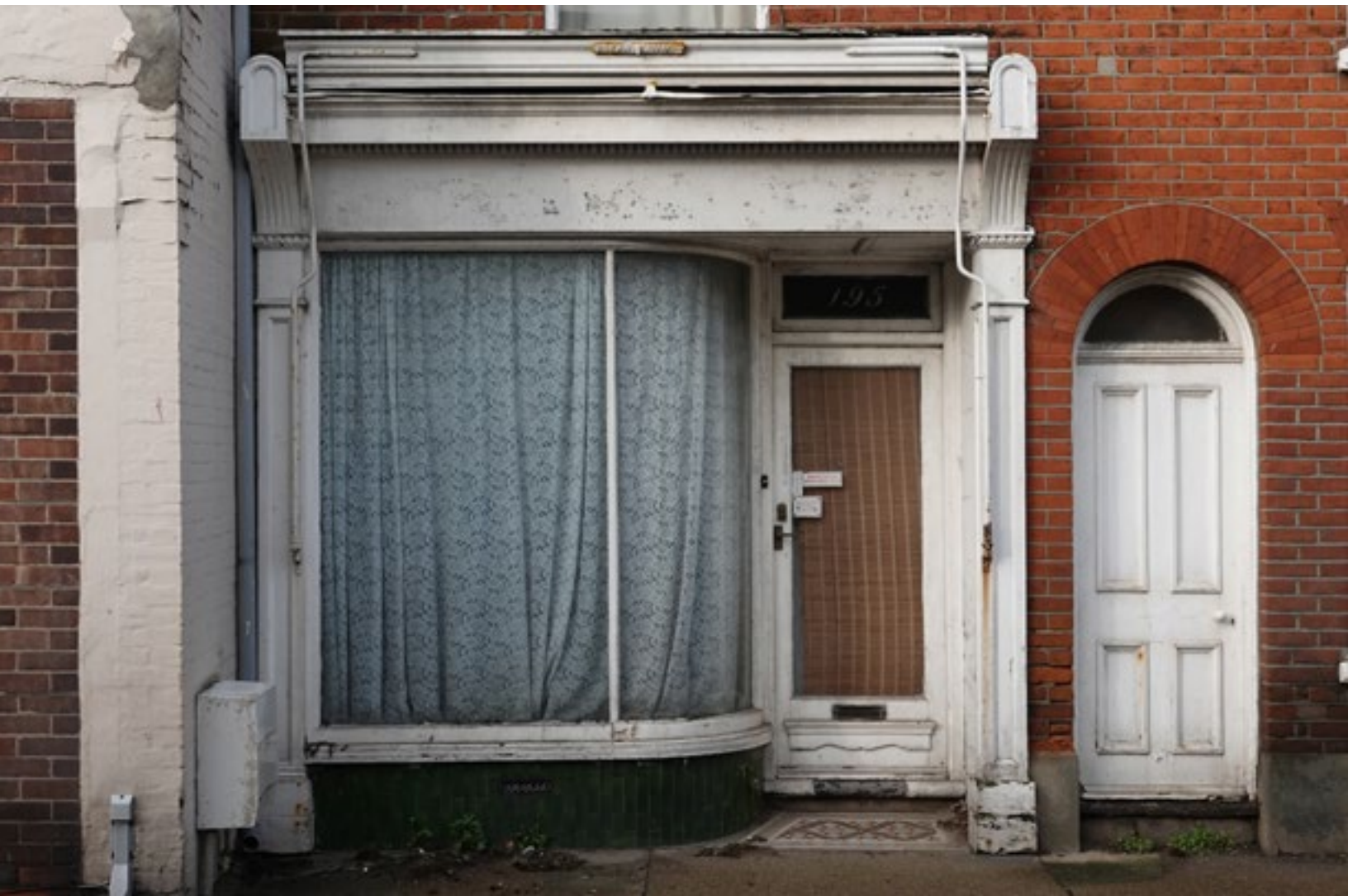
Fig. 043 Traditional timber shopfront with curved glass window. High Street, Gorleston
