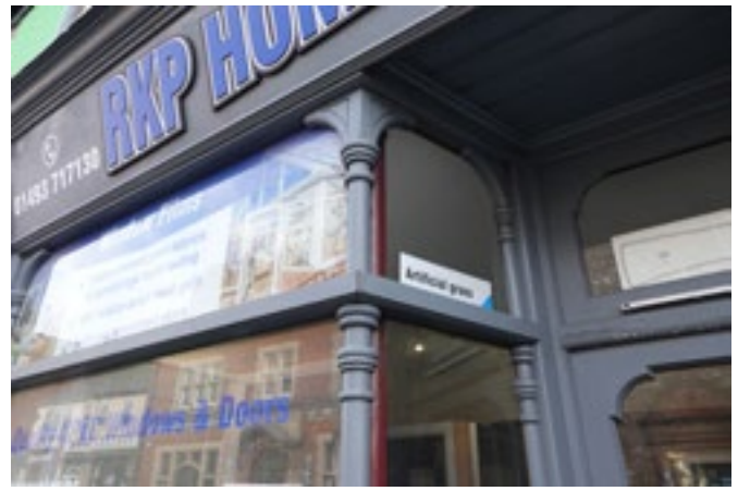
Fig. 030 Colonnette mullions with spandrels. Gorleston
