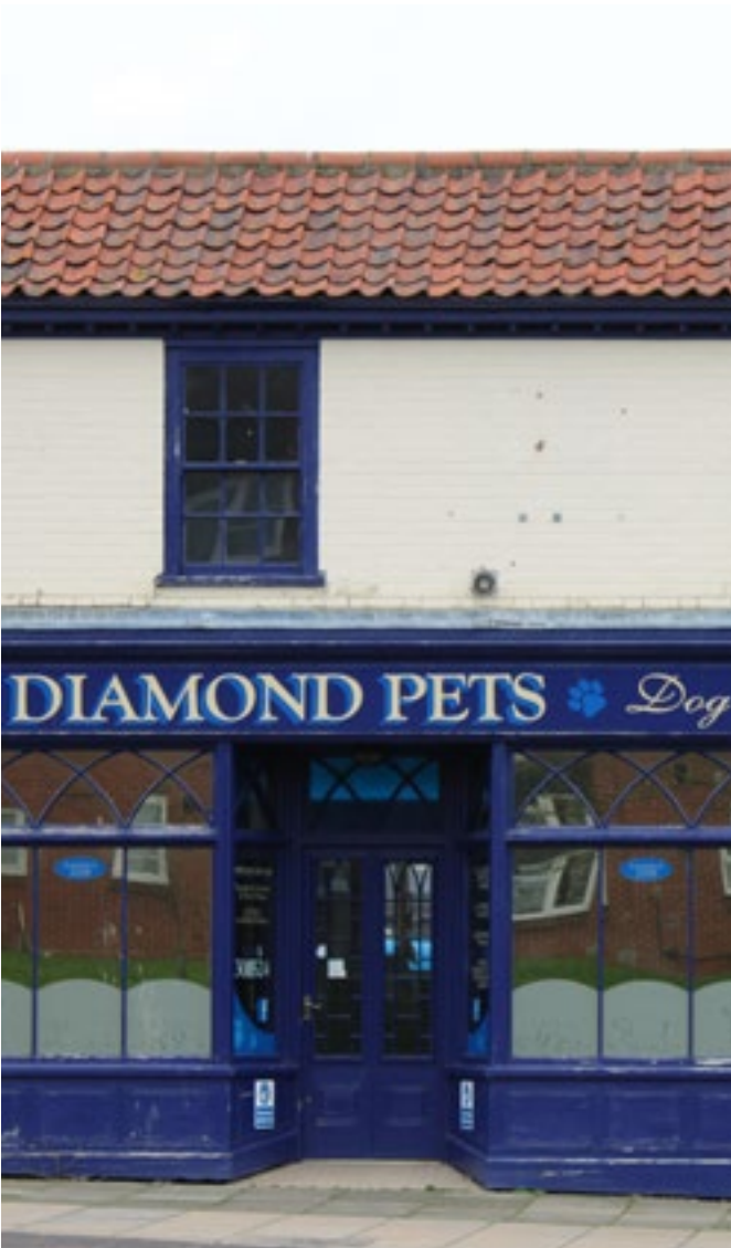
Fig. 035 Shopfront entrance - recessed doors with fan-light in line with the transom lights.
