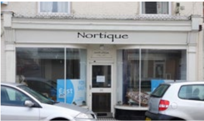
Fig. 039 Fascia angled towards the street - a traditional approach.
