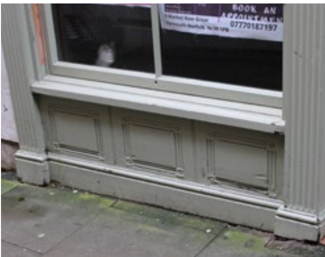
Fig. 027 Timber panelled stallriser
