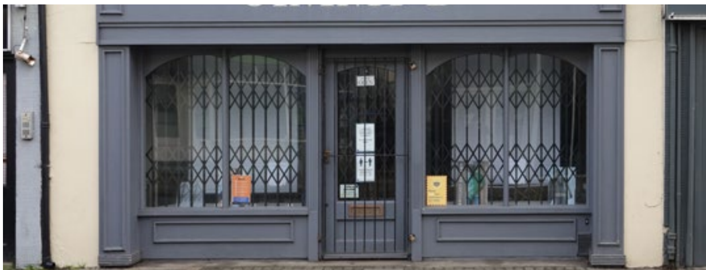
Fig. 048 Internal open lattice grilles.
