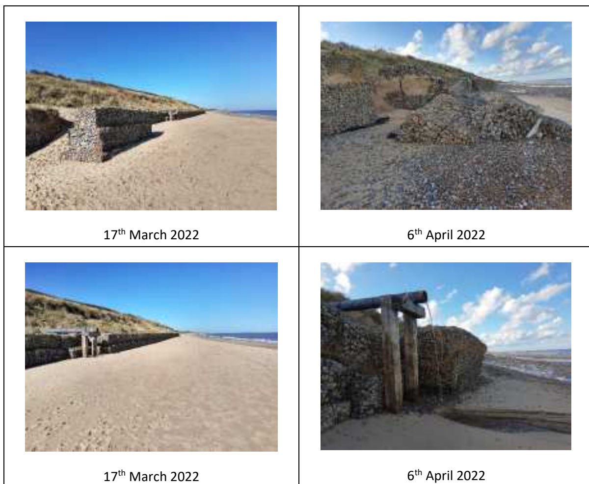
Figure 3 Lowering of beach levels and subsequent damage to Scratby gabion structure, March 2022 to April 2022
