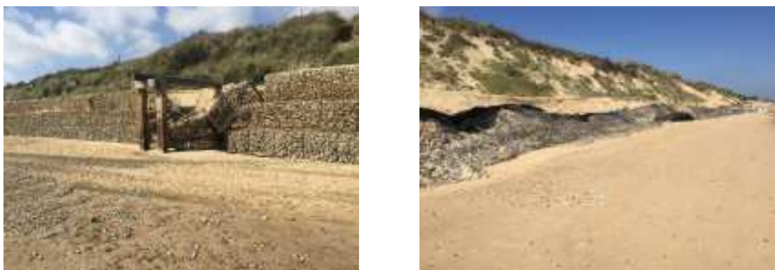
Figure 1 Previous damage to Scratby Gabions following the Spring 2018 'Beast from the East'
