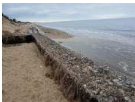
North-West of Damaged Gabions 19th May 2022
