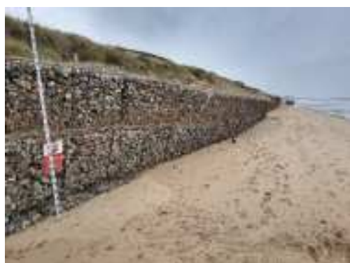
Figure 4 Forward rotation of the Scratby gabion structure, following the storm event of the evening of 31st March and 1st April 2022.
