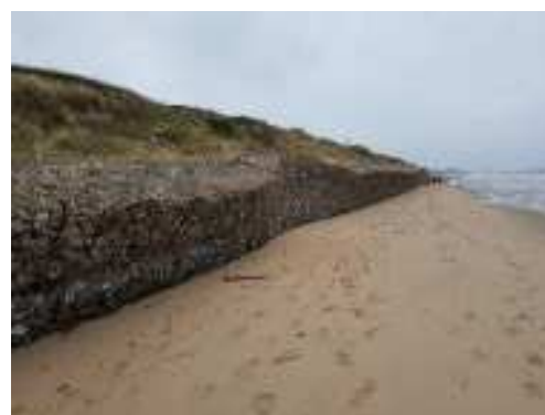
Figure 4 Forward rotation of the Scratby gabion structure, following the storm event of the evening of 31st March and 1st April 2022.
