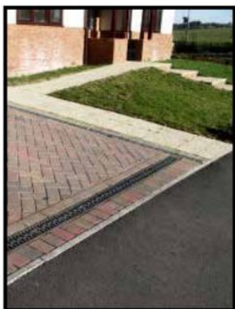
Positive example of drainage channel as demarcation of thresholds of water run-off from and to dwellings
