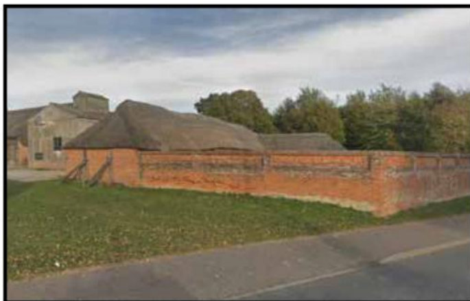
Traditional brick boundary wall
