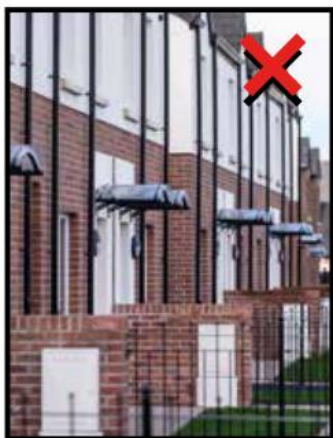
Poorly located meter boxes, their presence clutters front elevations
