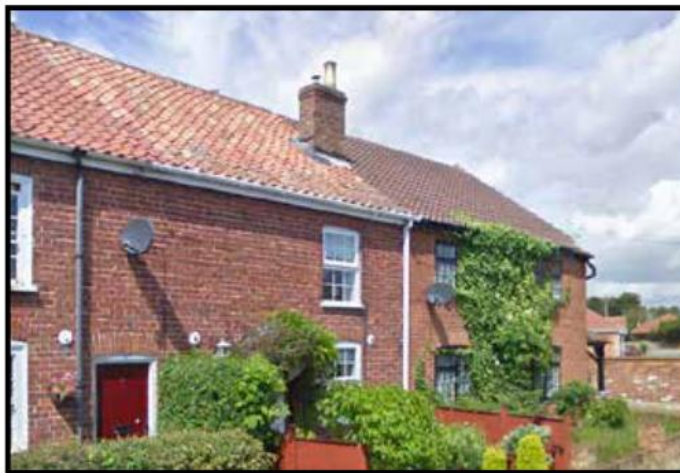
Brick facades and ceramic tiled roofs
