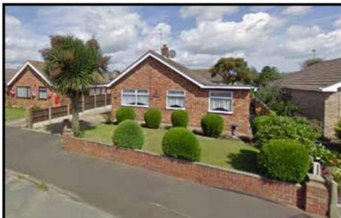
Low brick boundary wall
