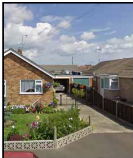
Common Rr. On-plot parking in garage
