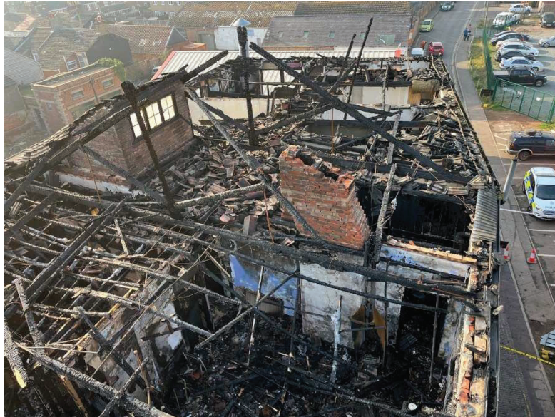
Figure 5 – High Level View of the Fire Damaged Central Roof & Second Floor Area Looking North
