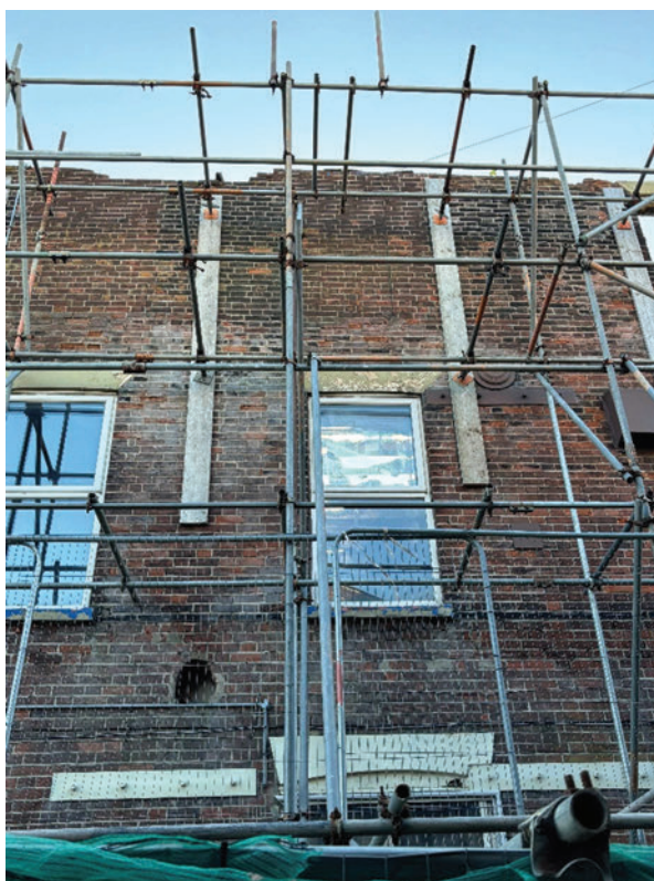
Figure 11 – View of Side Wall Showing Lateral Restraint Temporary Scaffold System and Localised Loss of Masonry at High Level
