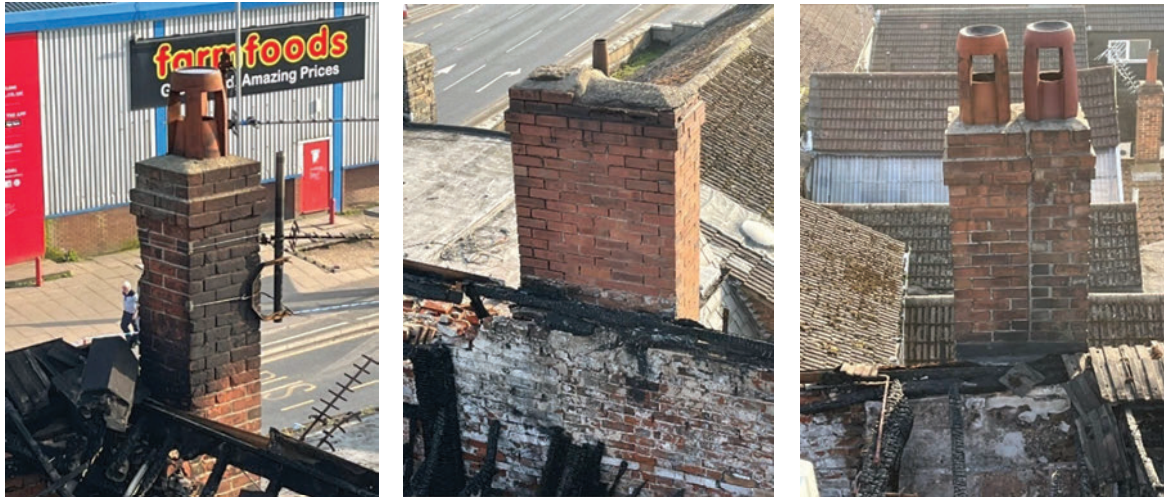
Figure 13 – High Level Close-up Views of Chimney Stacks on Party Wall Line (Photos taken on 24 th March 2022)
