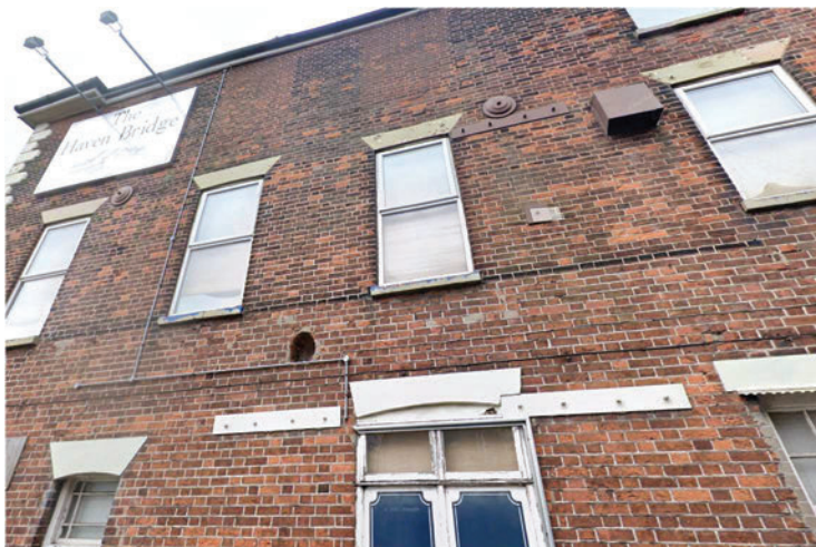
Figure 3 – East Facing Flank Wall of Haven Bridge PH showing Lateral Restraint Remedial Works Tie Rods and Pattress Plates at First Floor & Second Floor Levels
