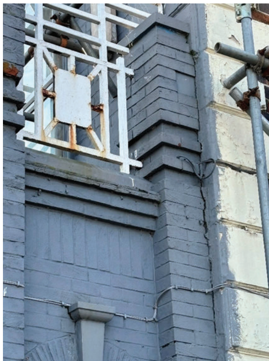
Figure 10 – Vertical Cracking at Junction of Single Storey Front Projection with Front Elevation of Main Unit
