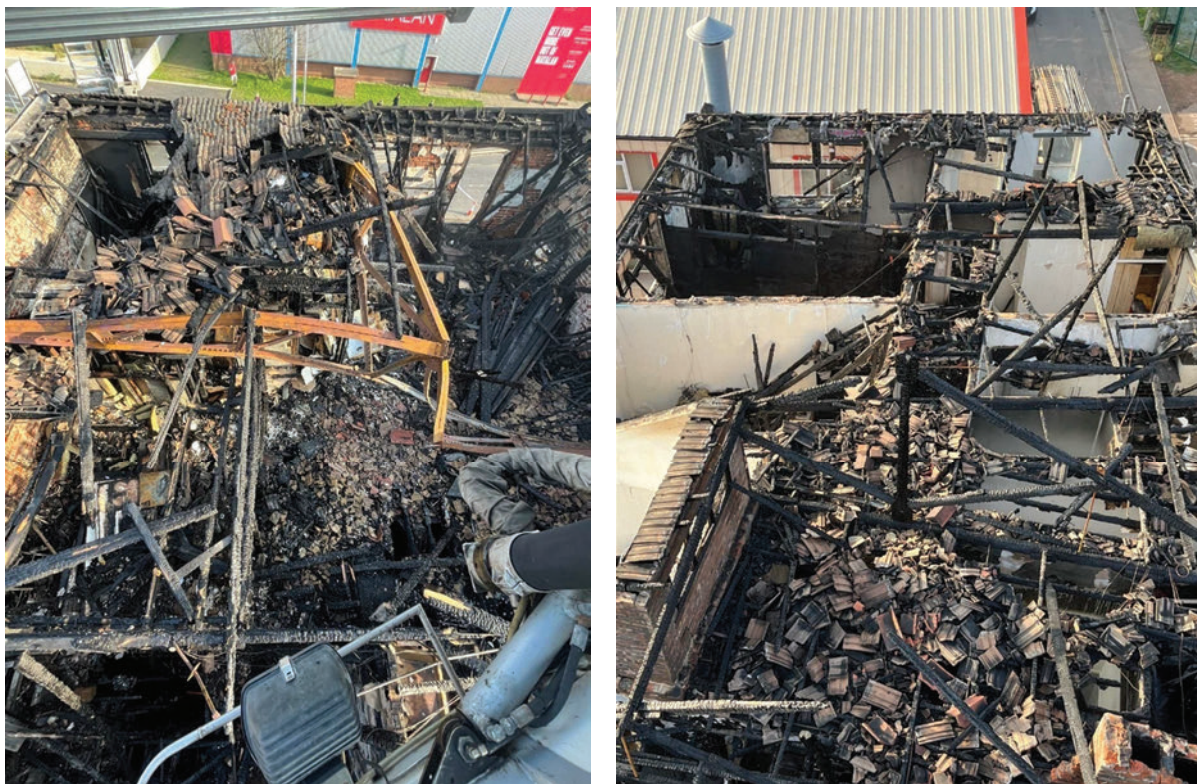
Figure 6 – High Level Views of the Fire Damaged Roof & Second Floor Looking South (left) and North (right)
