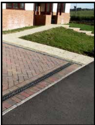
Positive example of drainage channel as demarcation of thresholds of water run-off from and to dwellings
