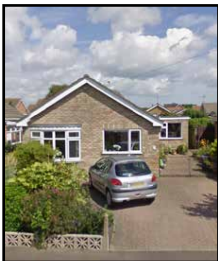
Common Rd. On-plot parking on driveway
