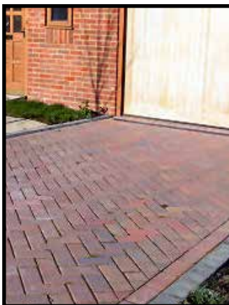
Positive example of drainage channel as demarcation of thresholds of water run-off from and to dwellings
