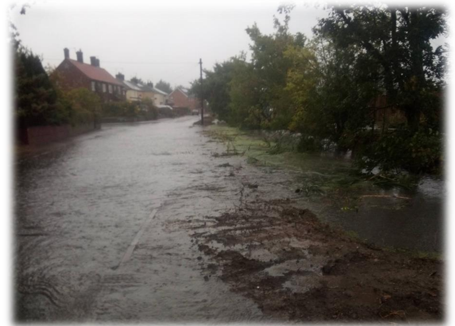
Flooding, Rollesby Road, November 2019
