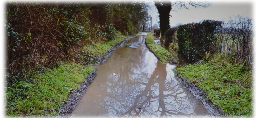
Flooding, Marsh Road, January 2021
