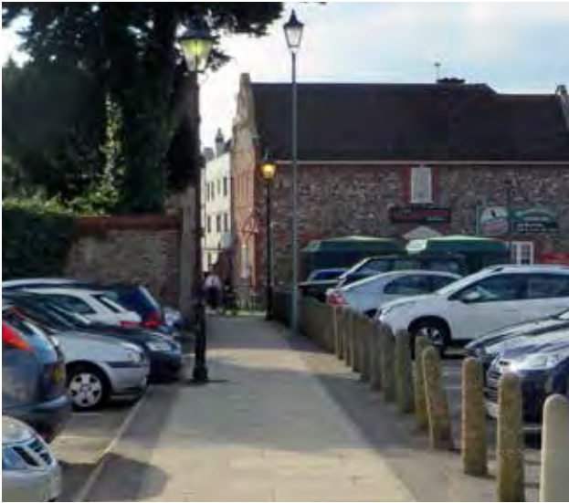
The Mariner's Tavern on Howard Street viewed from Palmers' carpark, where the paving and lighting of Row 60 is continued through the carpark to link from Market Place to Hall Quay
