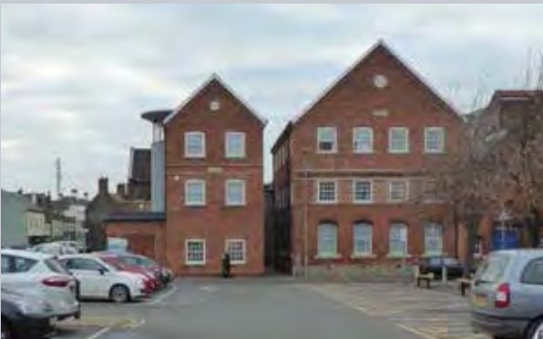
View westwards through the two blocks of Lighthouse Medical Centre divided by Row 83
