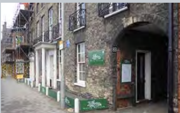
Row 83 entry at Elizabethan House, South Quay
