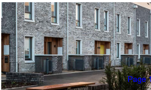
Fig. 41. Examples of well designed air source heat pump screening at Marmalade Lane, Cambridge. Architect: Mole Architects
