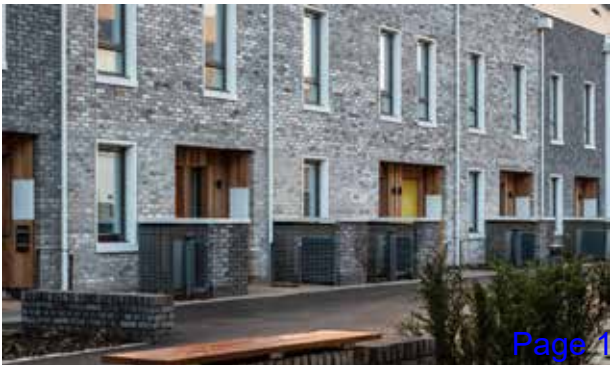
Fig. 43. Examples of well designed air source heat pump screening at Marmalade Lane, Cambridge. Architect: Mole Architects
