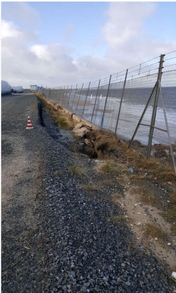
Figure 1-5 - Rotation of the wall (06/04/2020)
