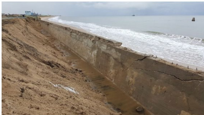
Figure 1-7 - Remedial works to relieve pressure on the landward side of the wall (23/09/2020)
