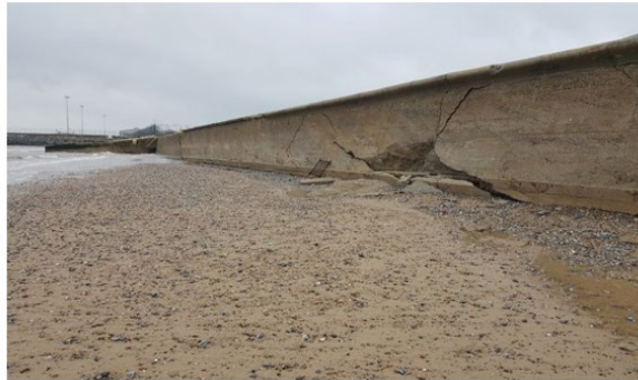
Figure 1-6 – Cracks formed on the wall (16/02/2021)
