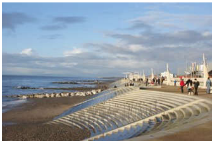
Figure 5-2 - Indicative stepped revetment structure [10]
