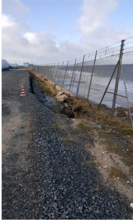
Figure 1-5 - Rotation of the wall (06/04/2020)
