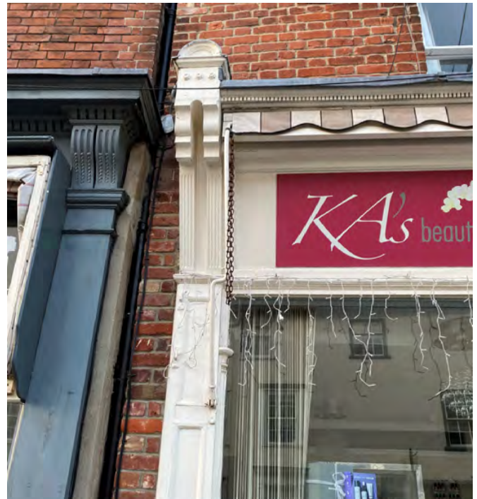
Fig. 055 Integrated blind box with a sprung roller housing a retractable canvas awning. Metal arms allow the blind to extend out and storm chains prevent movement.
