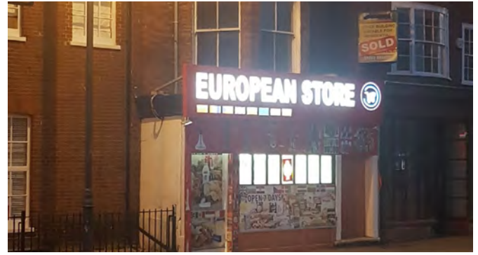
Fig. 051 Internally illuminated box-type fascias should be avoided, especially if they are bulky, with full-face illumination and are crudely bolted-on over the existing fascia board.
