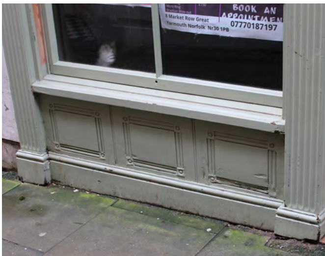
Fig. 033 Timber panelled stallriser.
