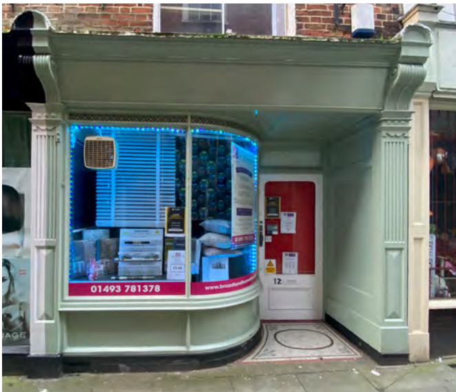
Fig. 032 Timber panelled stallriser.
