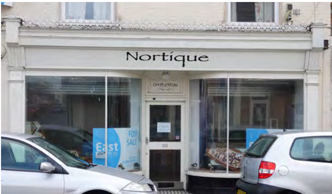
Fig. 044 Hand painted lettering onto the fascia board is the most appropriate form of fascia signage.
