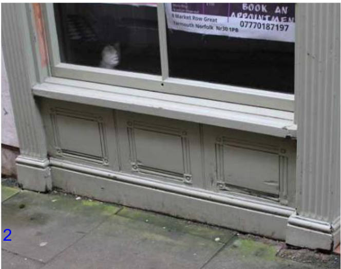
Fig. 033 Timber panelled stallriser.
