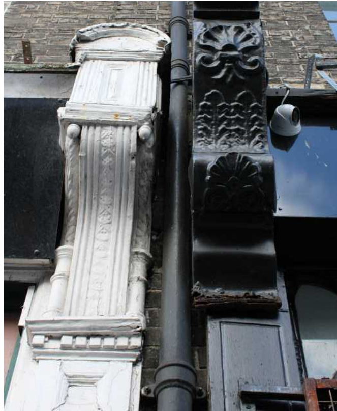
Fig. 048 Victorian console brackets.
