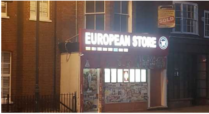
Fig. 051 Internally illuminated box-type fascias should be avoided, especially if they are bulky, with full-face illumination and are crudely bolted-on over the existing fascia board.
