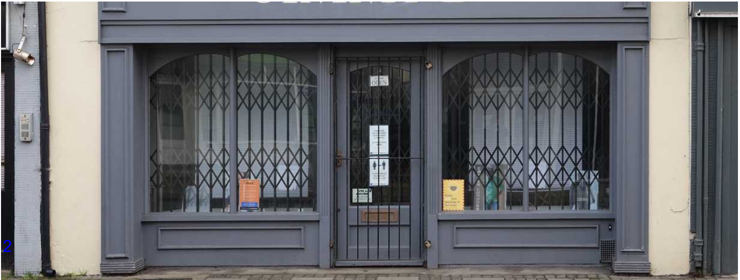
Fig. 054 Internal open lattice grilles.
