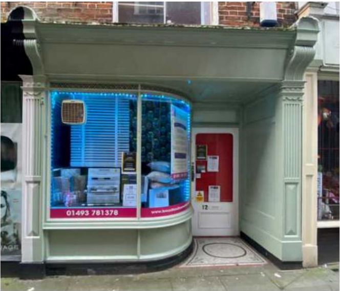
Fig. 032 Timber panelled stallriser.
